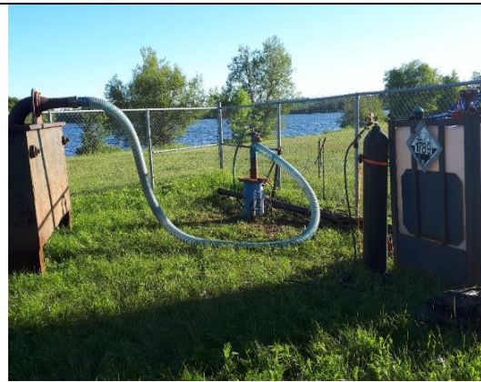
Photo 6: General Rehab Setup at Well 7
