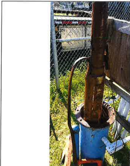
Photo 5: Pump Removal
