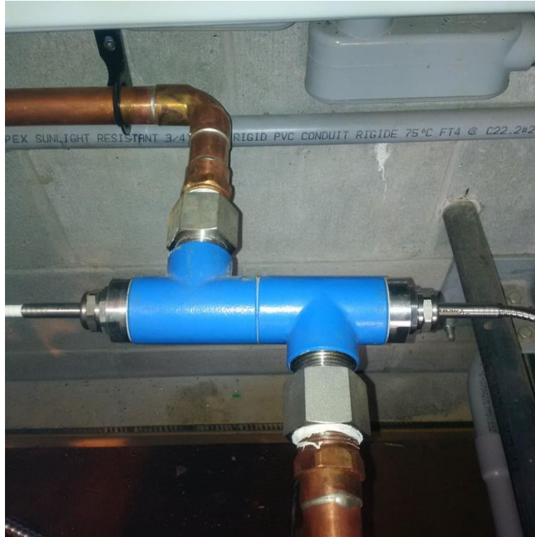
The in-line colour sensor flow cell
